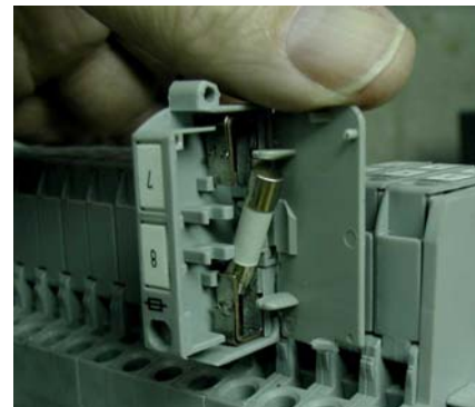
Figure 3-10b, Fuse Replacement
